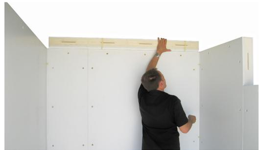
6. Slot the ceiling support brackets into the edges of the ceiling panel/s.
