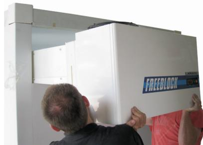
2. Ensure the refrigeration unit is fully inserted and flush with the interior wall surface.
