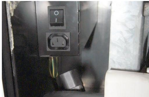
4. To reassemble, reconnect the mains isolation plug and switch on, locate the front panel onto the support brackets at the bottom of the cabinet opening and push the bottom brackets into the bottom of the cabinet to lock in place, and refit the return air grille.
