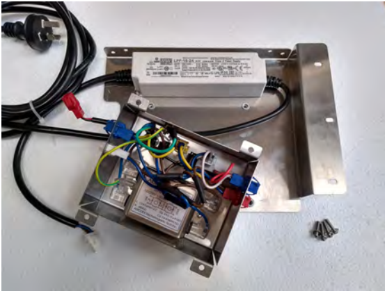
GN1/1 underbench cartridge electrics box
