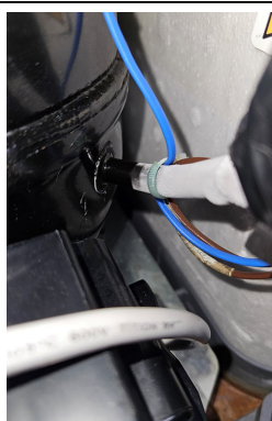
Correct frost back at 20°C
