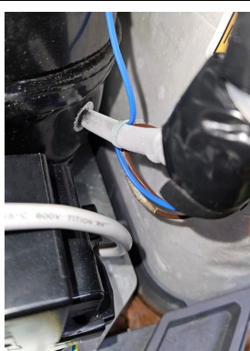
Correct frost back at 10°C
