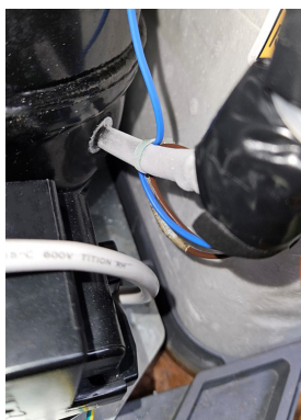
Correct frost back at 10°C
