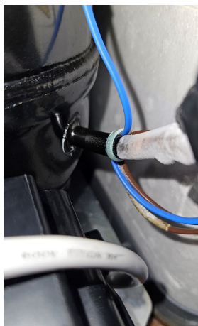
Correct frost back at 30°C
