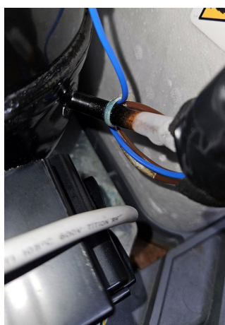
Correct frost back at 40°C
